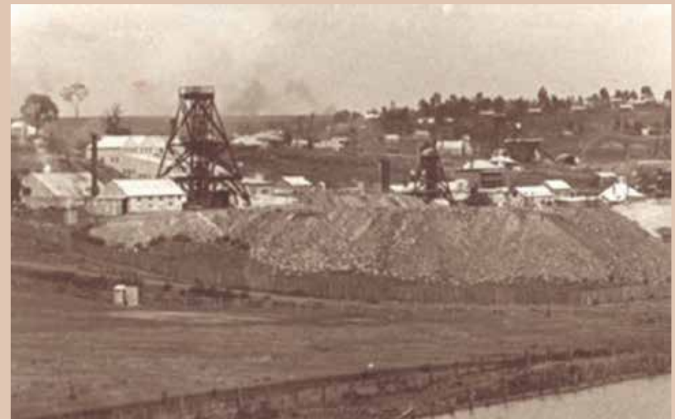
Wentworth and Reform Shafts looking southwest, showing the extensive waste rock dumps. (Source: Sheridan Collection, Mitchell Library)
