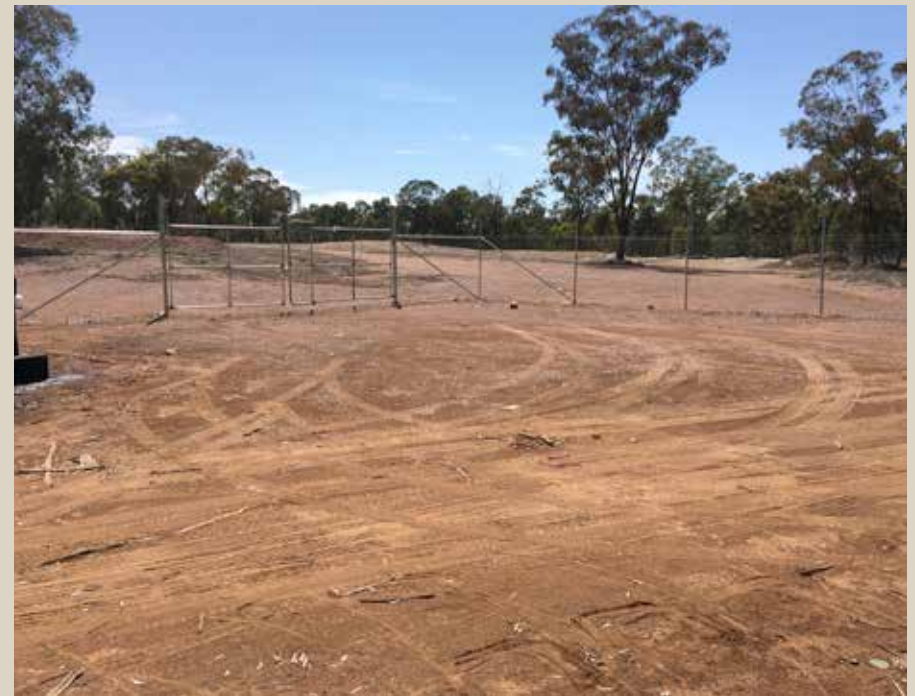
Closed landfill site, Fifield.
