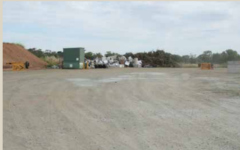
Nyngan Waste and Resource Recovery Facility Levelling of Existing Site for Recycling Drop off Area, February 2016
