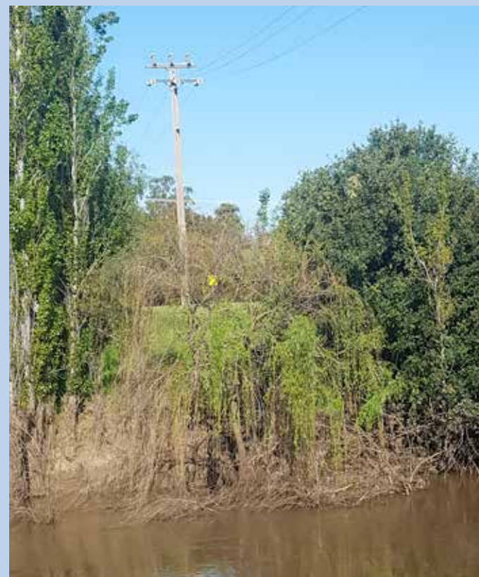
Mature Willow Tree directly drilled, located at Warren Town Bridge
